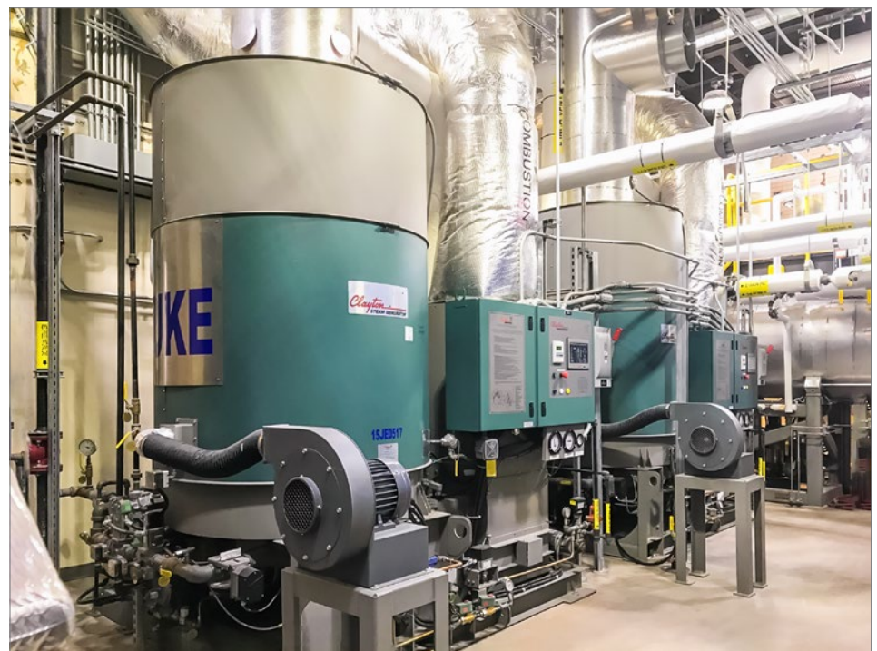
Two Clayton steam generators and horizontal condensate receiver skid (in background)
