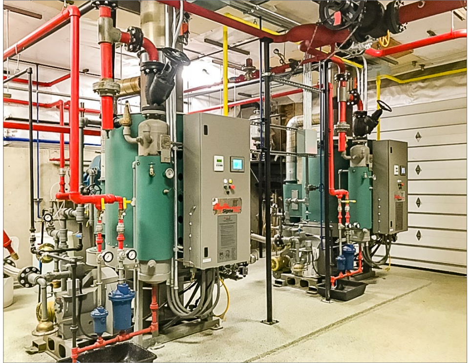
With the fast reaction time of Clayton 150 BHP generators, steam could be produced on demand for morning production. That resulted in an immediate 32+% energy savings.
