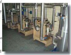
An added advantage of the vertical configuration of the Clayton Steam Generator is that the heat exchange surfaces can be easily cleaned by flushing with water from top to bottom under gravity. Over time, certain light deposits from the recovered fat can form on the coil surface and it is possible to carry out the cleaning process very effectively and quickly using this method. On other boiler designs it would be necessary to perform a complete drain down which would produce a large water loss.
