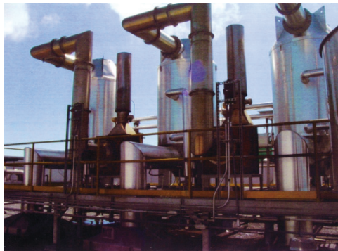
Steam generators, an essential part of a heat recovery system, capture gasses that would be exhausted and use that heat for boiler systems.
