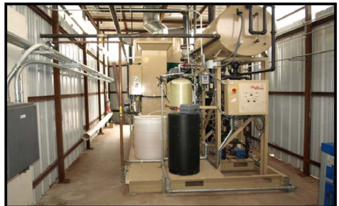
Feedwater components on packaged skid
