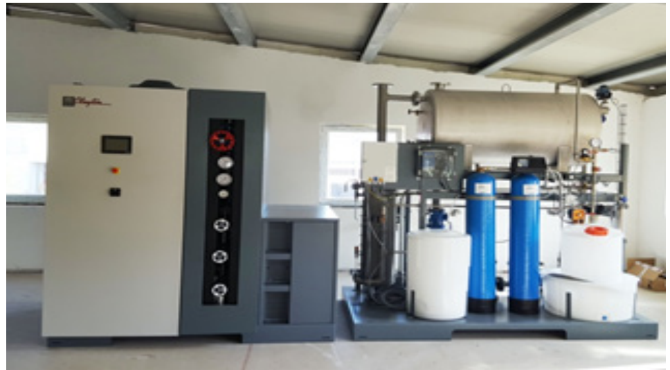
The compact design of the Steam Master made it an ideal fit, along with its optional water treatment package, which includes a stainless steel tank, and integrated chemical dosing system and a double filtered dehumidifier.
