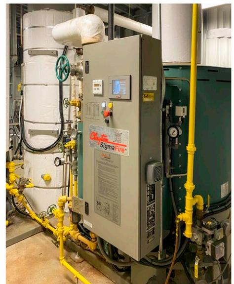
SigmaFire SF50 Steam Generator 50BHP: The unit’s compact size and low weight is ideal for the Seaside Farm building and meshes well with the FMT food processing equipment.
