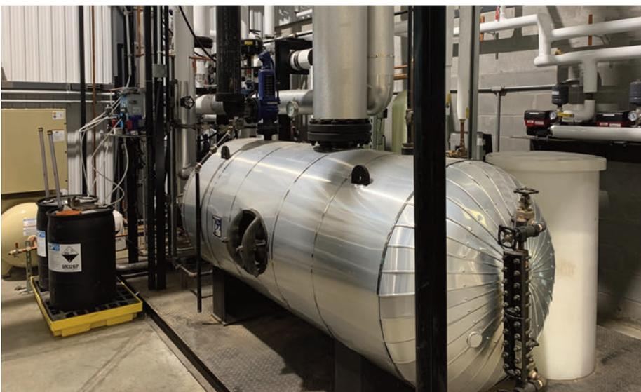
Powered by the new, more efficient Clayton Industries boiler and specially designed accumulator, the autoclave at Daniels Health in Brampton, Ontario, Canada, began operating a whopping 25% faster.
