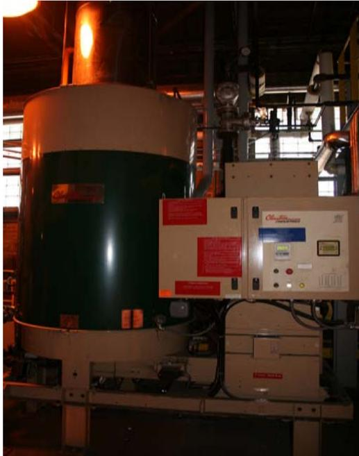
Clayton 250 BHP Steam Generator equipment on coke oven gas in Europe, but did not have installation in the US. With the operator issue out of the way, Joe Magni could concentrate on the combustion issue. Clayton Senior Sales Engineer, Mike Sabol provided Joe with drawings of the Clayton cog burner used in Europe. Since the design used large opening and high velocities the potential for fouling is minimized.
