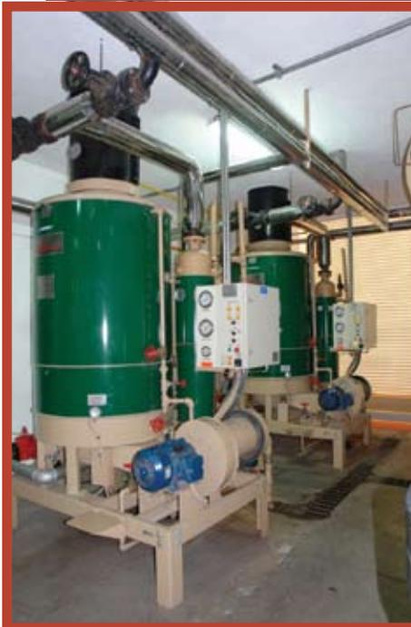
In the boiler room of Nicro Bolta, Puebla, Mexico, the new system incorporates two, 185 BHP steam generators, a 5,000-liter tank with heat exchanger to deliver 230°F (110°C) water, and a speed-controlled pumping system that ensures proper pressure at discharge points.
