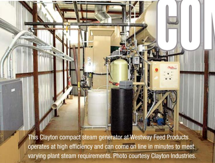
This Clayton compact steam generator at Westway Feed Products operates at high efficiency and can come on line in minutes to meet varying plant steam requirements. Photo courtesy Clayton Industries.
