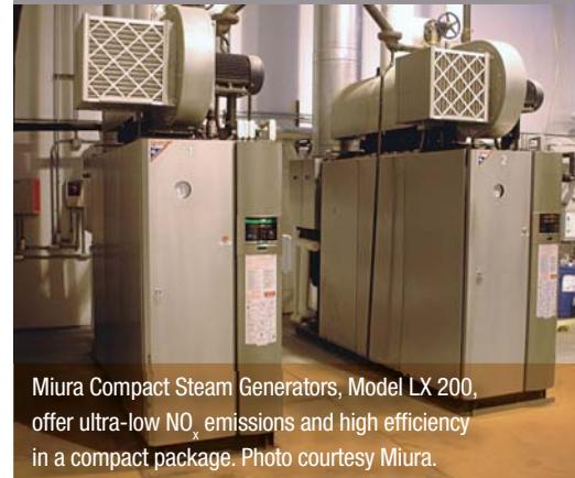
Miura Compact Steam Generators, Model LX 200, offer ultra-low NO<sub>x</sub> emissions and high efficiency in a compact package. Photo courtesy Miura.
