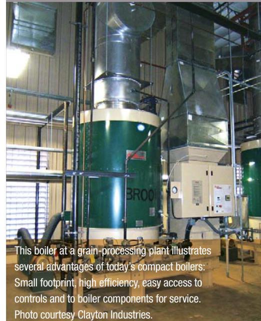
This boiler at a grain-processing plant illustrates several advantages of today's compact boilers: Small footprint, high efficiency, easy access to controls and to boiler components for service. Photo courtesy Clayton Industries.
