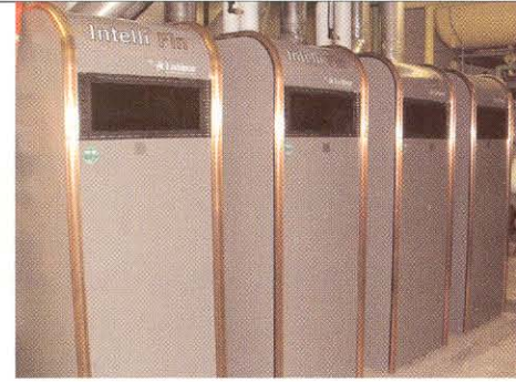
Zero sidewall clearance design of the Lochinvar boiler allows multiple units to be installed in a very small space.
