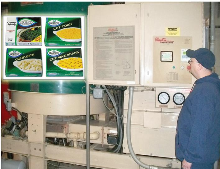
▶ Wes Seabrook stands next to the PLC-based controls of the Clayton Steam Generator, which provides steam on demand for processing Seabrook Farms' vegetables. Inset: Seabrook frozen products have been around for decades.
