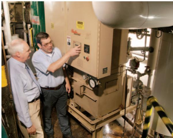
Clayton's Mike Sabol and Marzetti's Maintenance Manager Jerry Hoffer fine tune operation of the Clayton EG-304-1-DZ steam generator, a once-through, forced-flow, water-tube boiler that utilizes a steel, helical-coil heat exchanger. Source: Clayton Industries.
