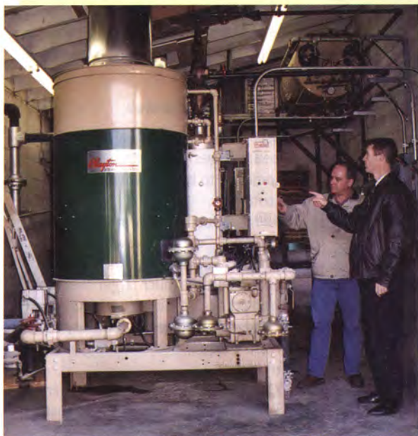
Black Rock Milling's Scott Kamper, left, and Chip Maguire of steam generator supplier Clayton Industries at the control panel of one of the Le Grand, CA., feed plant's twin 100-hp, high-efficiency, mono-tube coil steam generators, used to supply steam for pelleting and flaking operations.
