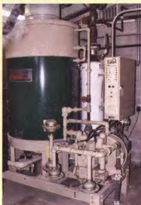
Black Rock Milling's Scott Kamper, left, and Chip Maguire of steam generator supplier Clayton Industries at the control panel of one of the Le Grand, CA., feed plant's twin 100-hp, high-efficiency, mono-tube coil steam generators, used to supply steam for pelleting and flaking operations.
